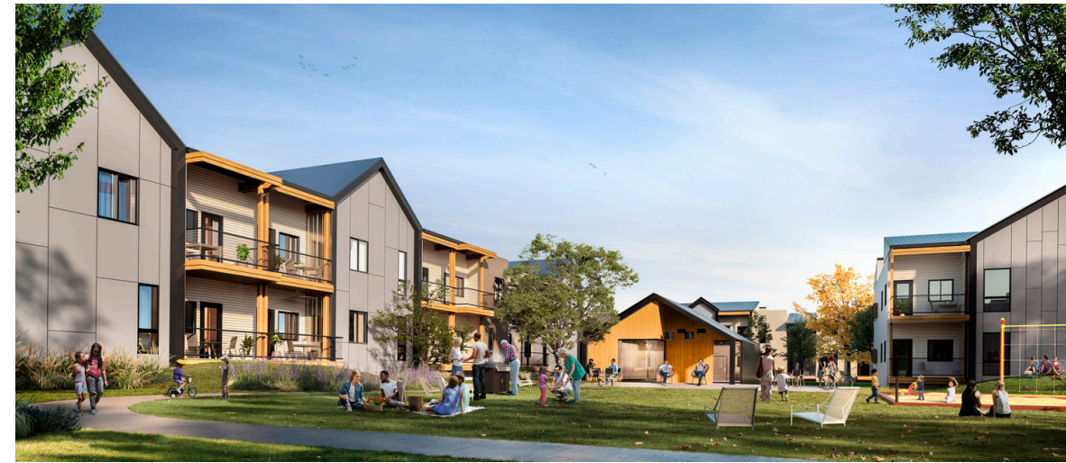
(L) (R) Greenfield Commons is the largest modular affordable multi-family project in California at over 200 units. HED acted as Architect of Record and designed the project, which is targeting net-zero.
